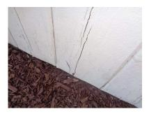
Combination of Stucco, Wood shingles, CONDITIONS, Attention: The wood siding was damaged/deteriorated. These conditions are conducive to moisture intrusion/deterioration. Repairs or replacement needed.
